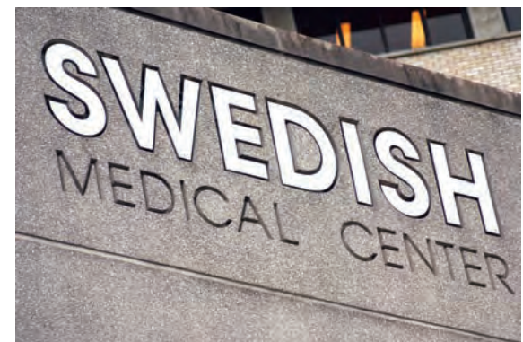
Swedish Medical Center installed an innovative heat exchanger that is saving 5,000 gallons of water per day.
