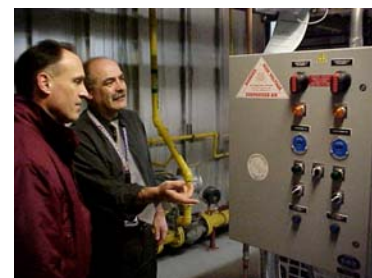
Cornell Amaya of SPU and Tom Nance, Chief Engineer of Group Health Hospital, inspect a new medical air compressor that replaced a once-through liquid ring compressor.
