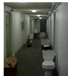
Toilet replacement in progress at the 55-unit El Nor Apartments in Seattle.
