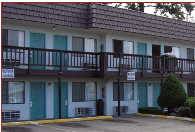
The Sea Tac Valu Inn in Highline Water District replaced toilets, showerheads and faucet aerators.
