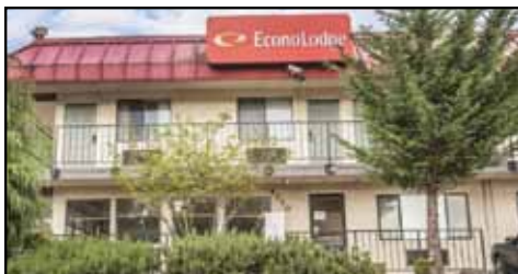
This hotel in Renton upgraded restroom fixtures and ice machines.
